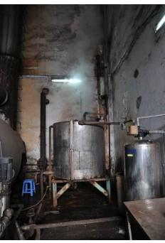
Open and no-insulation tank of condensed water
