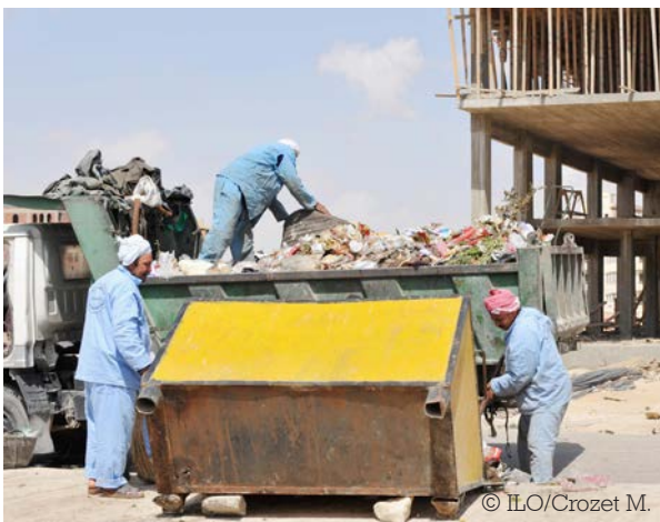
Figure 2.3.1. Rubbish collection on a construction site in the suburb of Cairo.
