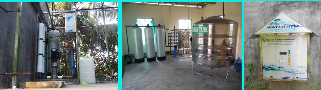
Process of Reverse Osmosis system installation and installed water ATM
