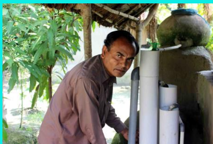
Local technique of water purification (Pond Sand and Filter_PSF_ system)
