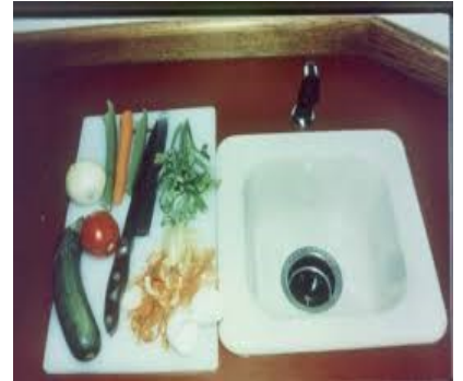
Separate Kitchen Organic Resource Sink with 1hp electric disposal plumbed to the Bio-Matter Resequencing Converter—Composting Tank
