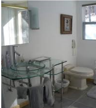
Dometic/SeaLand Ultra-Ultra Low Flushing Toilets plumbed to the Bio-Matter Resequencing Converter—Composting Tank
