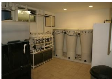
Bio-Matter Resequencing Converter, Greywater System and Enfinity Ozone and the first prototype Reverse Osmosis Disinfection and Filtration Recycling System
