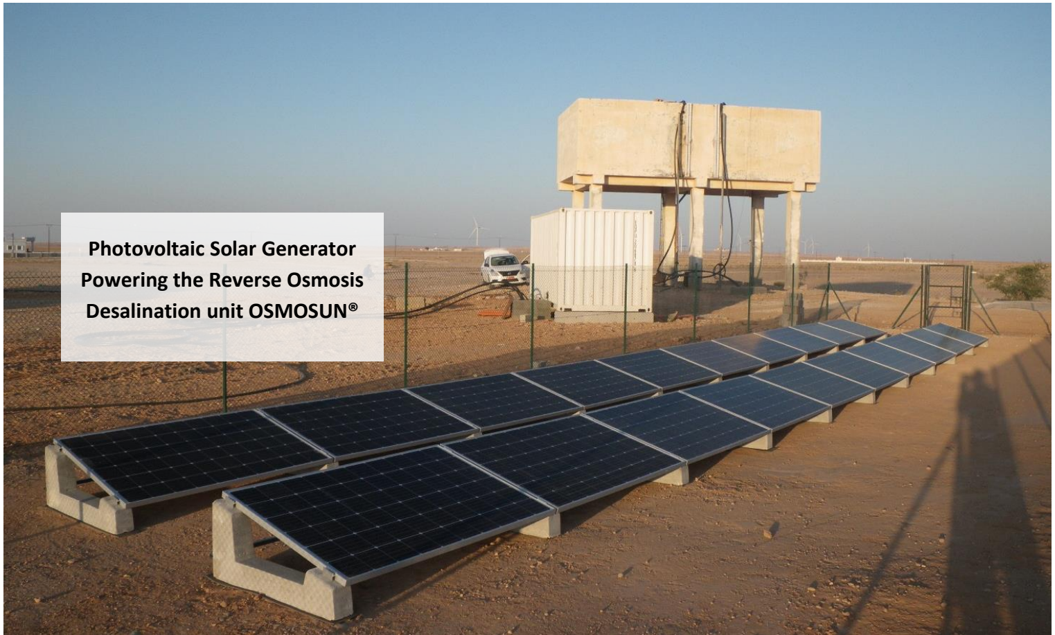
Drinking water daily production of 21m 3 powered by 100% solar energy
