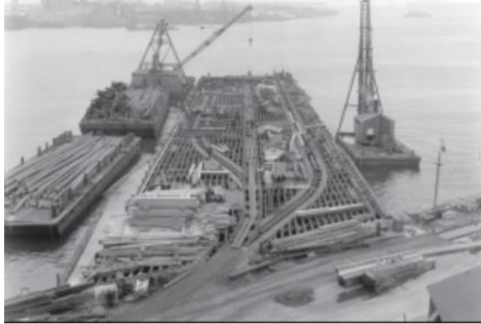
Figure 1- Original Pier 4A During Construction
