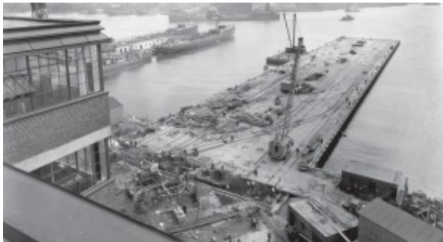
Figure 2- Pier 5 during construction
